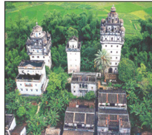
THE THREE TOWERS OF JINJIANGLI
